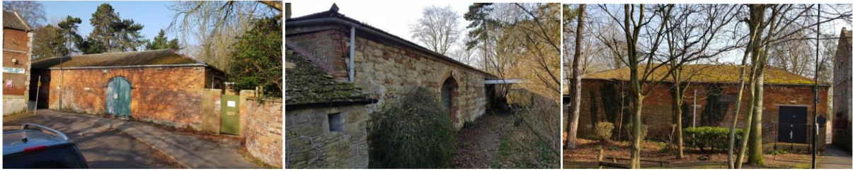
Photos 9, 10 and 11: Views of the curtilage listed C19 Woolstore Building (south, north and west facing elevations taken in February 2018). The Woolstore roof (1970s covering) is proposed for removal along with the upper parts of the external walls and all internal walls. An aperture of circa 5m will be created in the southern and northern elevations to create a principal vehicular access through to the rear garden area. The internal Woolstore area will provide 13 No. parking spaces, recycling and bin storage.
